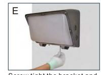
Screw tight the bracket and fixture.
